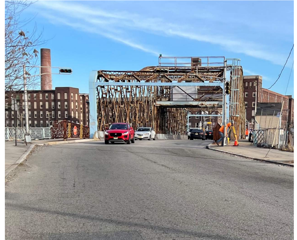
Substandard Angle Point and Lack of Shoulders
