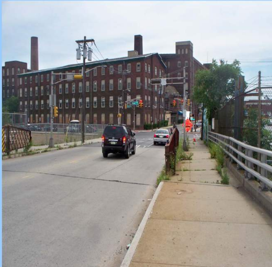
Photo 3: East approach to bridge looking east
