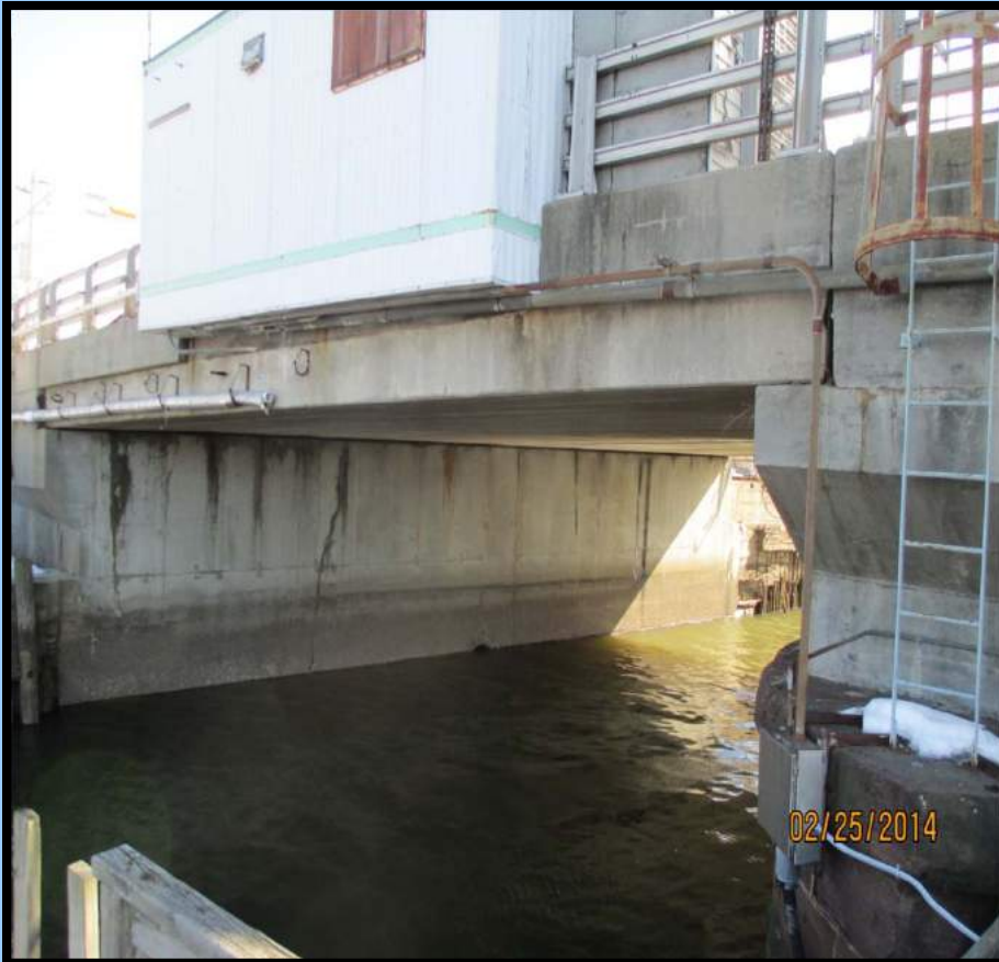
Photo 21: East approach span and east abutment
