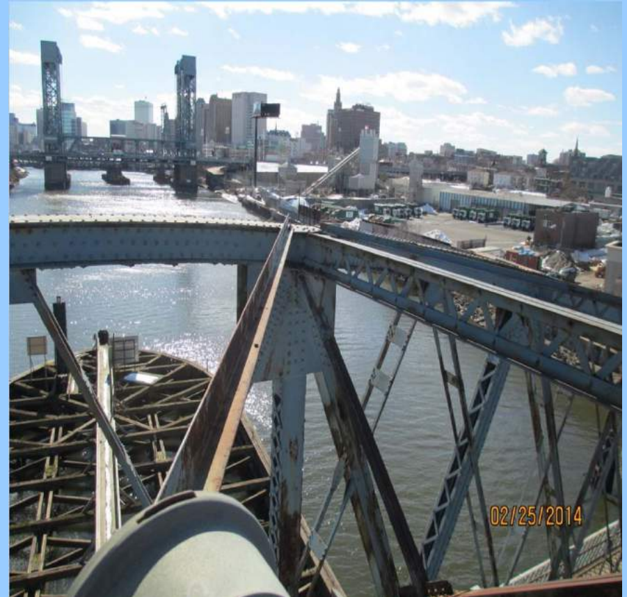
Photo 4: Looking downstream from bridge – I-280 Stickle Bridge in background
