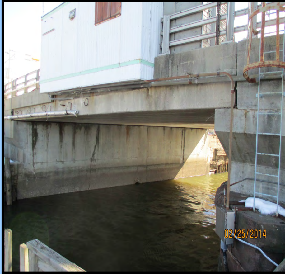
Photo 21: East approach span and east abutment
