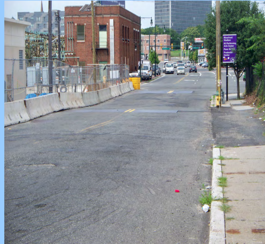
Photo 2: Looking west from bridge – note substandard outside shoulder width
