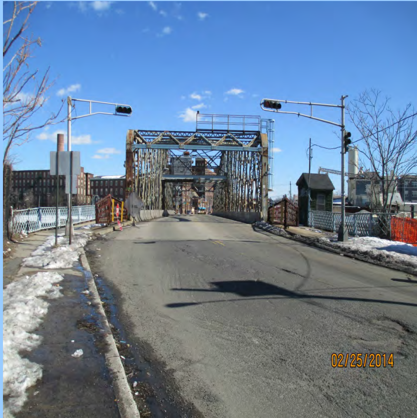
Photo 1: Bridge Approach Roadway Looking East – note substandard angle point
