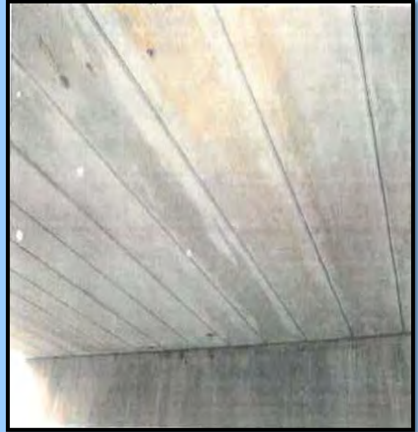
Photo 22: East approach span superstructure (pre-stressed concrete box beam)
