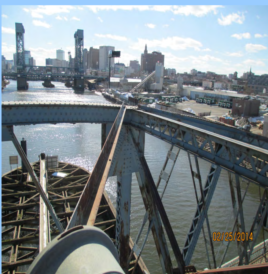
Photo 5: Looking south from top of bridge
