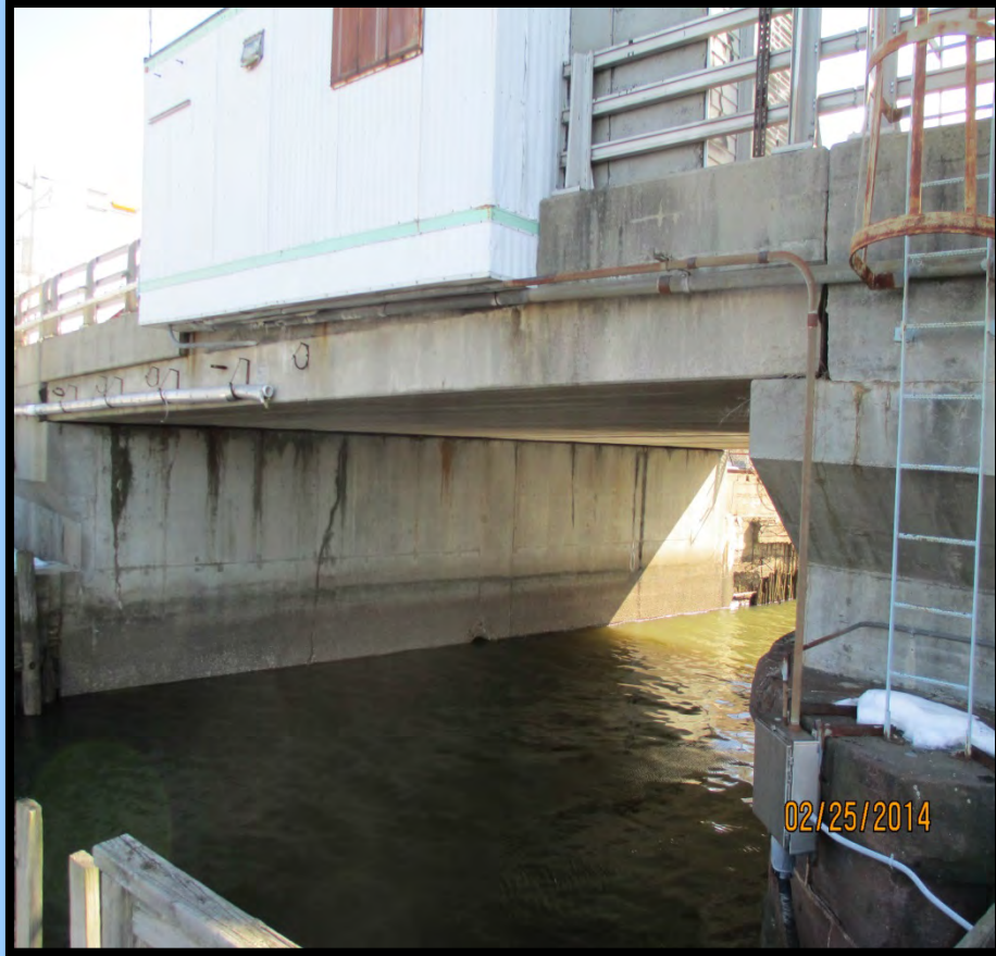
Photo 21: East approach span and east abutment
