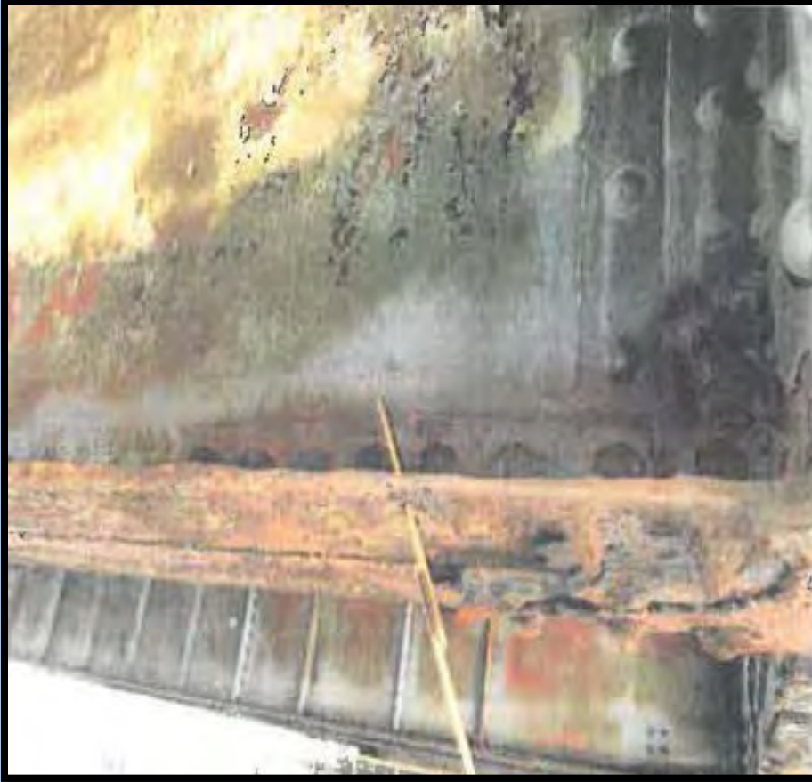
Photo 15: Severe rusting and hole in bottom flange angle leg of floor beam (FB12) of swing span
