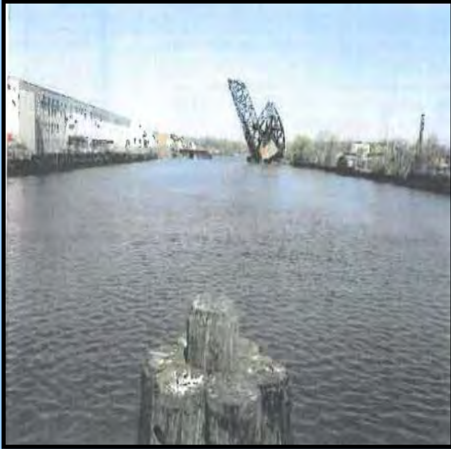
Photo 7: Looking north from bridge
